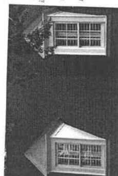
Do: The dormers on this fairly classical midrange building also have siding in the tympanum. Because this building is more refined than the first, the designer has used flush torque and goose siding to make the joints less apparent.
